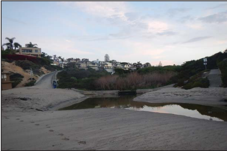
Photo 3: Facing north (upstream) at cement weir. Facing north.
