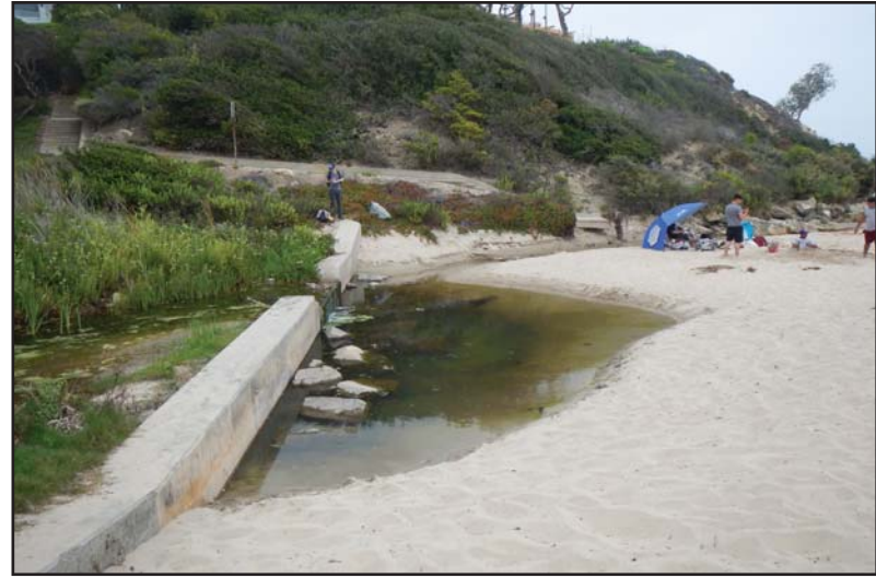
Photo 2: Profile view of cement weir. Facing east-southeast.
